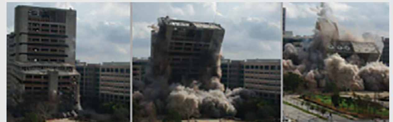
IMPLOSION OF MD ANDERSON CANCER CENTER IN HOUSTON, TEXAS
